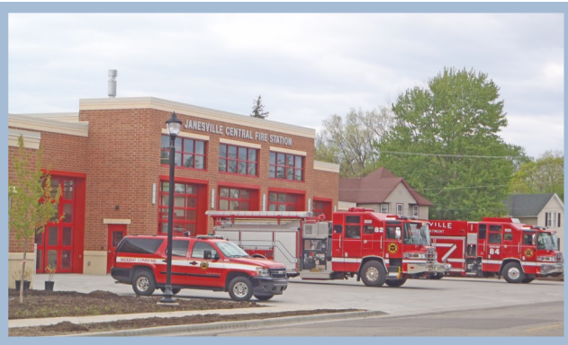
Construction of a new Central Fire Station was completed in the summer of 2016.
