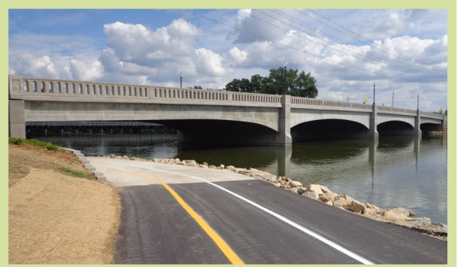
The reconstructed Jackson Street bridge opened to traffic on July 22, 2015. A bike path passes underneath the bridge's north side.
