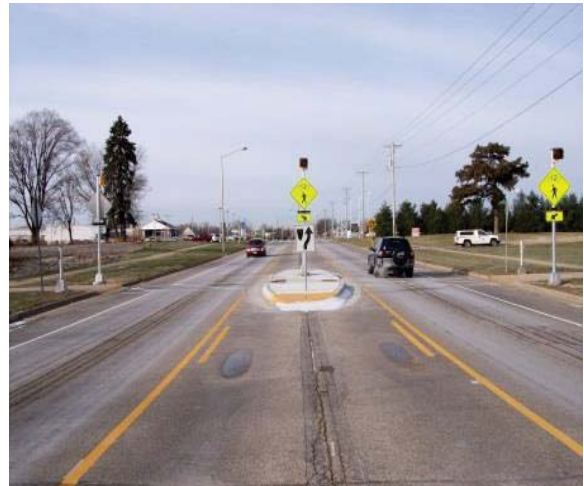
Safety improvement at E. Milwaukee Street and Ice Age Trail Crossing. Photo by MPO staff
