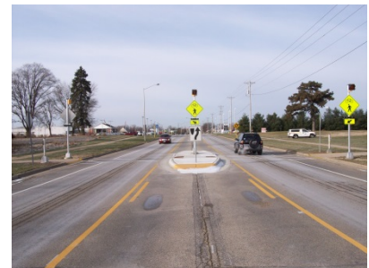
Safety improvement at E. Milwaukee Street and Ice Age Trail Crossing. Photo by MPO staff
