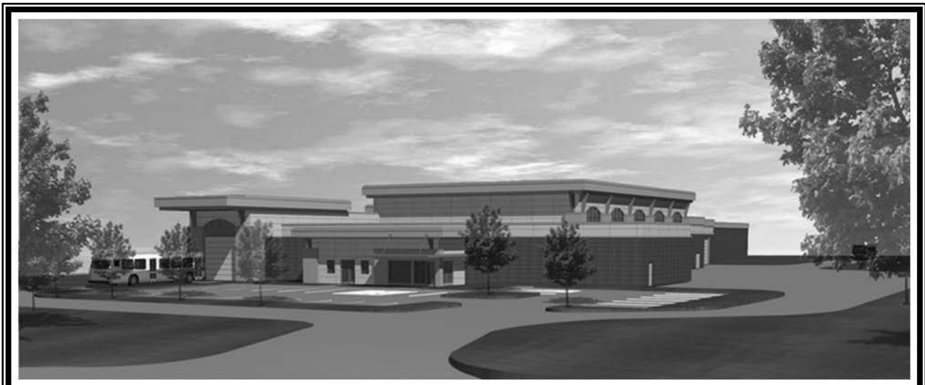
Transit Services Center photo by Angus Young & Associates
