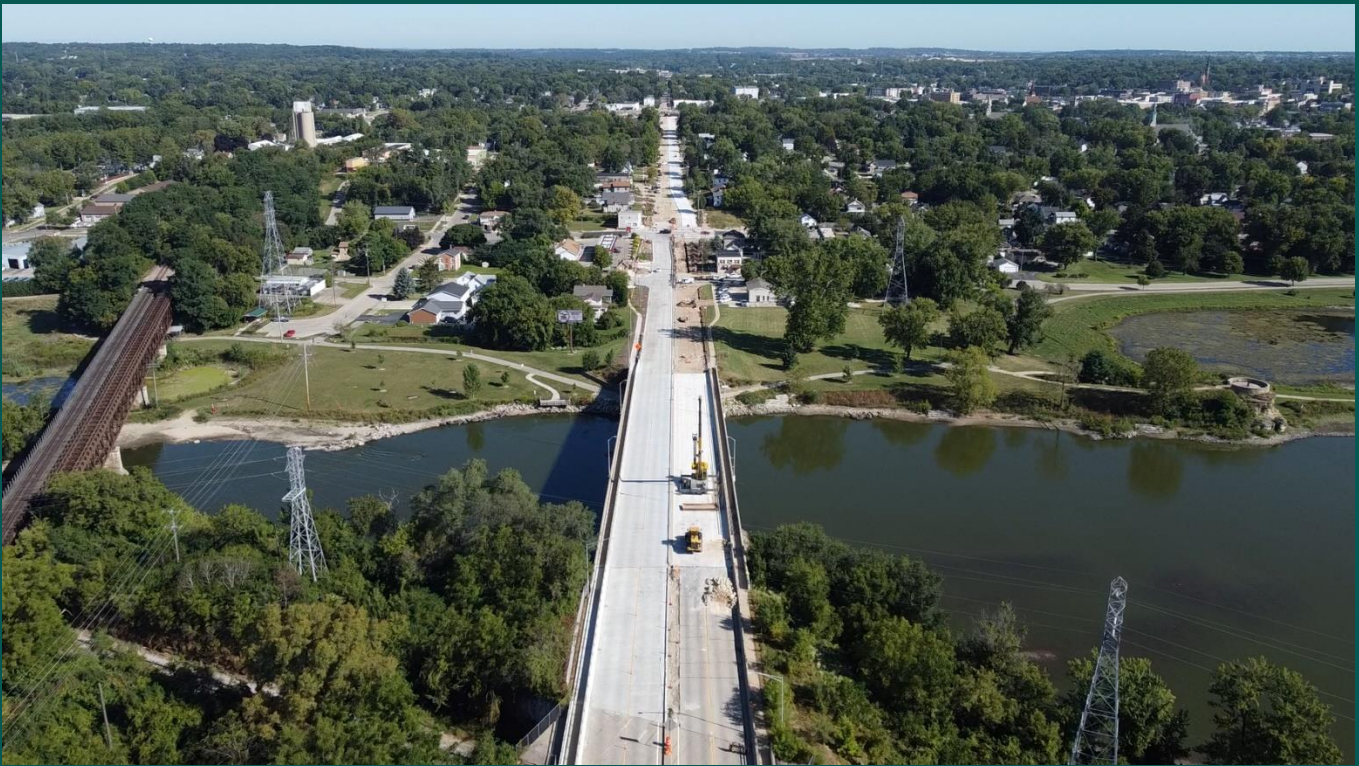
Center Avenue Bridge Resurfacing
