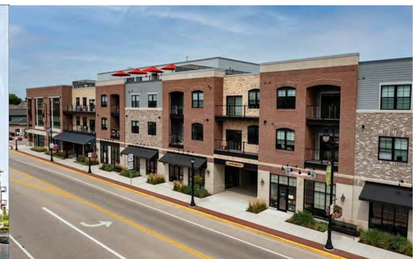
The Lamphouse is a mixed residential and commercial building in Waukegan, WI.
