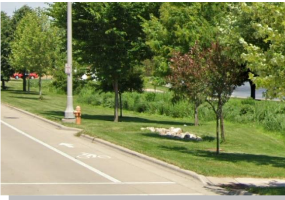
Bioswales, like this native plant rain garden along S River St, help to reduce flooding intensity and protect water quality in the Rock River.
