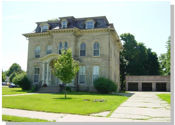
An example of Janesville’s stock of historically significant buildings.
