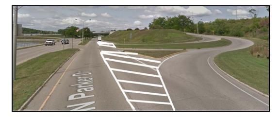
If the lane-drop suggestion is not feasible, then it is suggested that consideration be given to lengthening the EB to NB on-ramp to provide a parallel merging section and incorporating additional signing and pavement marking like suggestions #2 and #3 for the SB to WB ramp.
