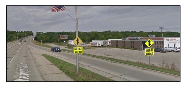
4. WB Memorial Dr., soon after the merge point with the SB to WB ramp from Parker Dr, an old turn-down guardrail end exists. It is suggested that consideration be given to updating the guardrail end to meet current standards and have a crash cushion. This is a **proactive** suggestion as there did not appear to be any guardrail collisions.
