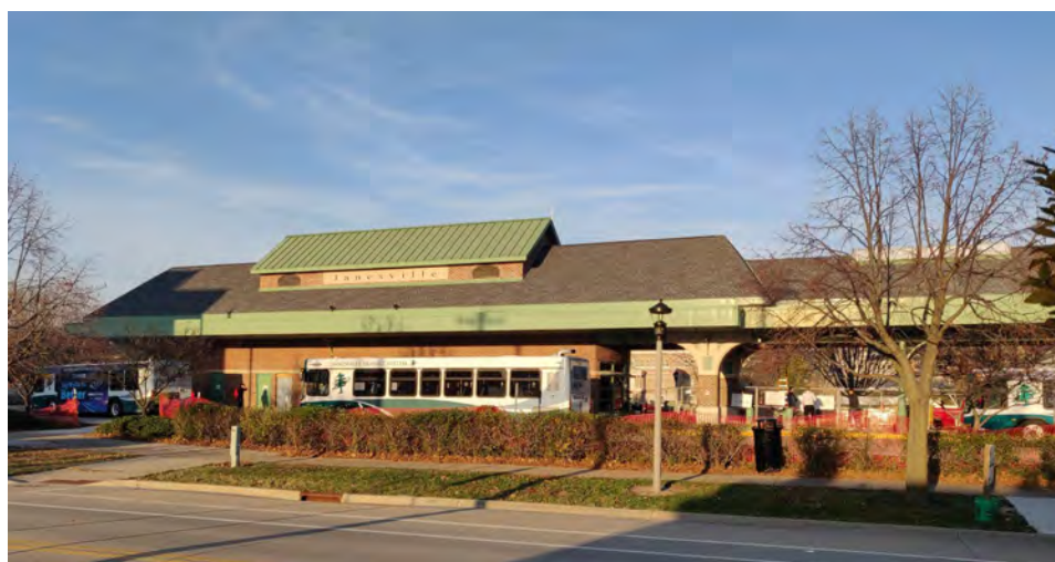
Figure 7. JTS Downtown Transfer Center
