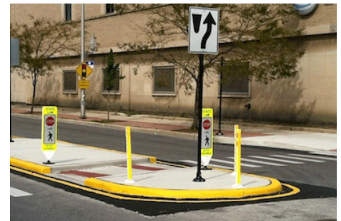
Median Refuge Island
